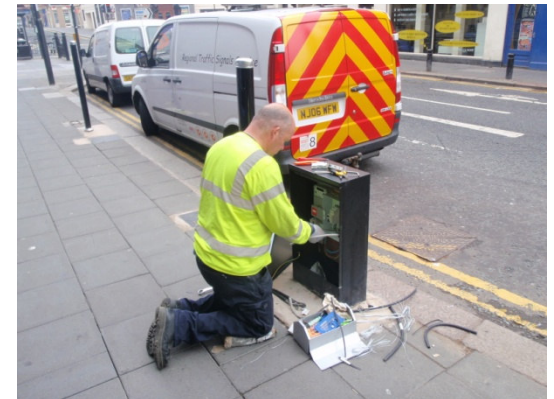
Charging point installation on Clayton Street
